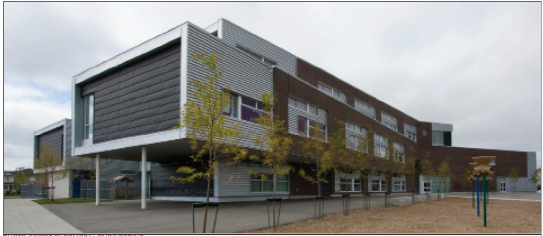
PHOTO CREDIT ENERMODAL ENGINEERING
